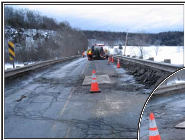
The first fix, on Monday, was to just get a very temporary cover on the hole.
