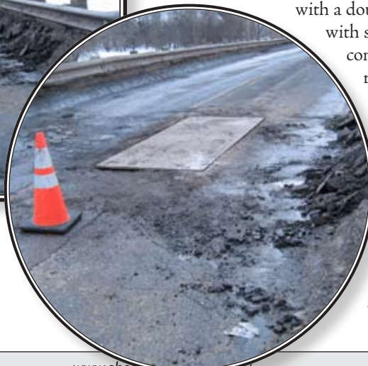
The first fix, on Monday, was to just get a very temporary cover on the hole.
